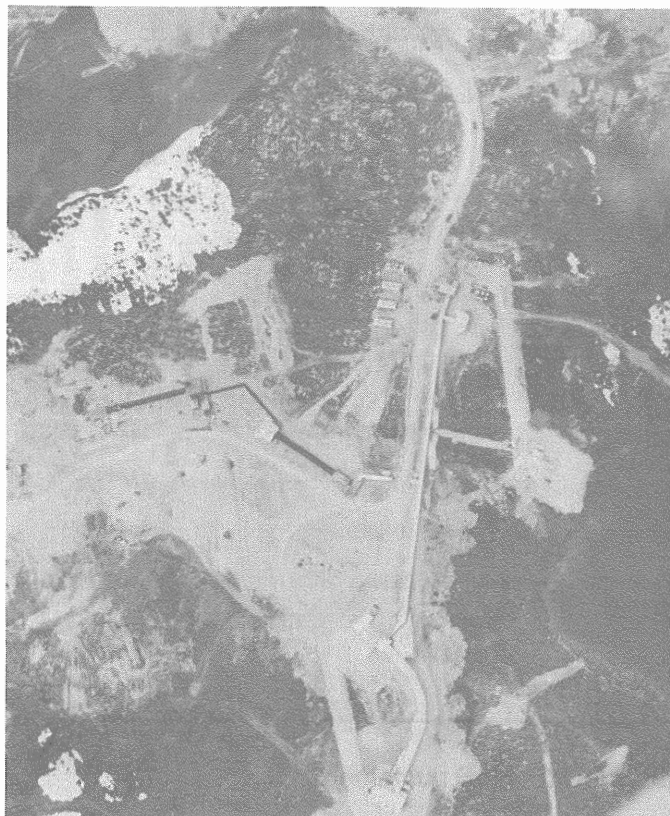
(a) Overall view.
