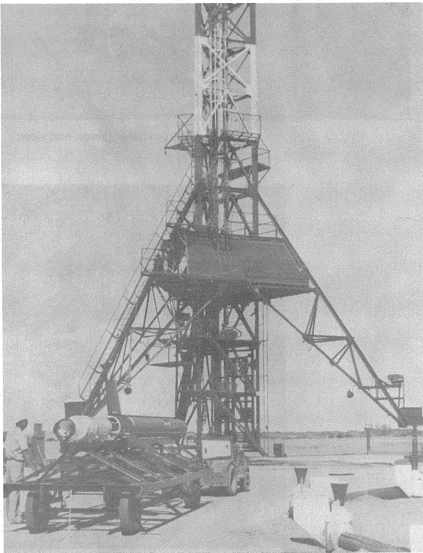
(f) Launch tower with sounding rocket ready for installation.
